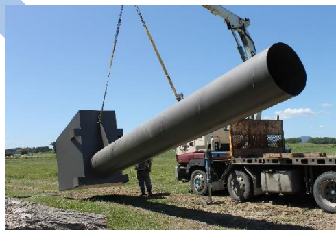
Installing floodgates
