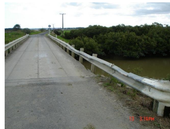
Te Kowhai Road bridge, Ruawai
