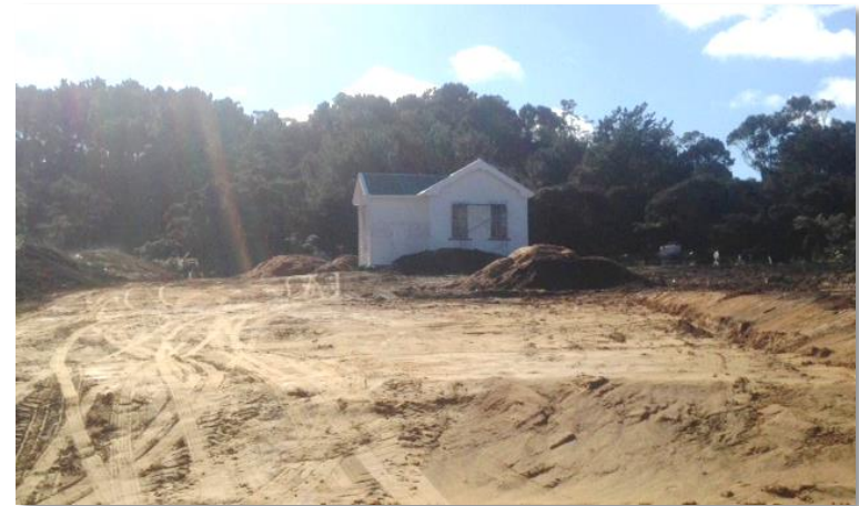
Relocating the old school house to Mangawhai
