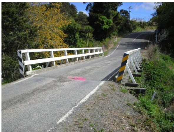
Bridge at Franklin Road Paparoa before replacement
